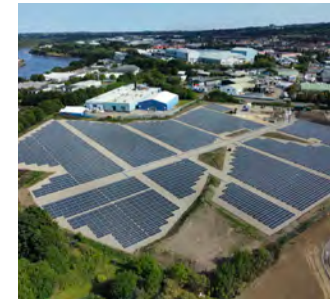
Solar Farm supplying GB Lubricants
